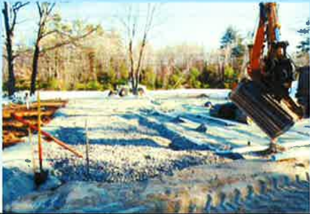
DAY TWO OF BED BUILD FUTURE VENT PIPE AT STAKE
