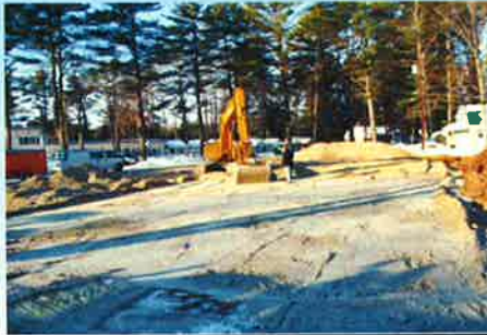
LEVELED WITH EXCAVATOR AND LASER
