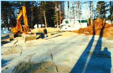
COVER STONE WITH LASER GUIDANCE FOR UNIFORM DEPTH AND TO BEAT 12" SNOWSTORM THAT NIGHT
