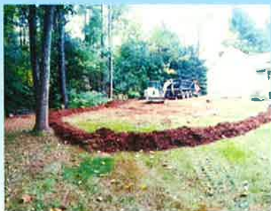
I NOW FAVOR EROSION CONTROL MIX AKA STUMP CHIPS
