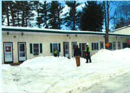
LOCATING BORING BY MOTEL FRONT- MAX DEPTH 18 FEET
