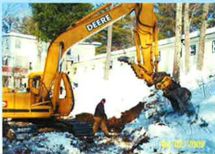
DUG A SMALL RECEIVING PIT ABOVE TANK AREA
