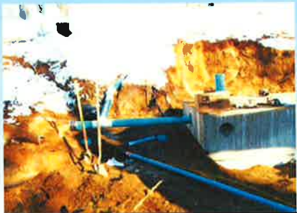
2" SDR CONNECTION TO PUMP TANK, PLUS TRACER LINE-UNDER SEWER LINES
