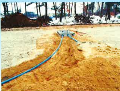
INSTALL FORCE MAINS
