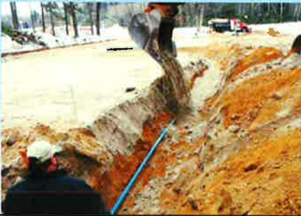
SDR PIPE BEDDED WITH SAND
