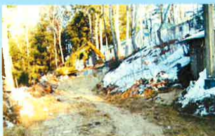
WORKING ON THE TWO "CABIN" TANKS
