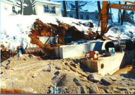
FIRST THREE TANKS
