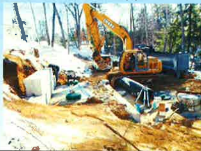
TANK AND RETAINING WALL CONSTRUCTION-STILL THREE MORE TANKS TO GO
