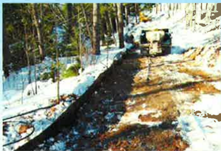
JANUARY 10 2009-SILT FENCE BELOW ZERO, WINDY
