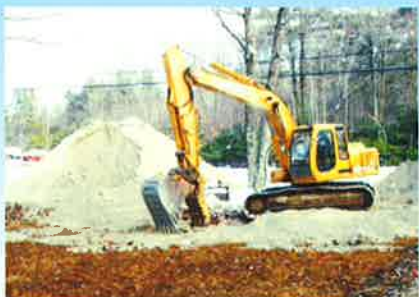
WASHED SAND IS PLACES AND MIXED INTO THE RIPPED RECEIVING SOIL
