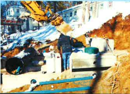
STEPPED TANKS REQUIRED RETAINING WALLS
