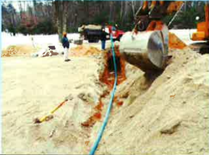
FORCE MAINS SLOPED TO PROVIDE DRAINBACK
