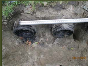
1.75 Ft. Center-to-Center Spacing Consistent Throughout
