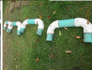
Raised Connections Constructed Properly
