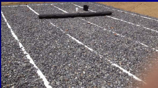
If more stone was to be added after inspection why is the fabric ready to roll out?
