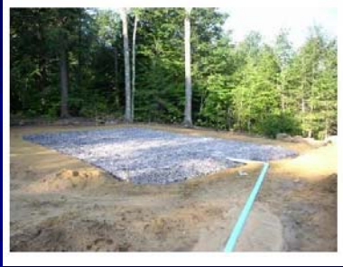
Stone and pipe excellent job
